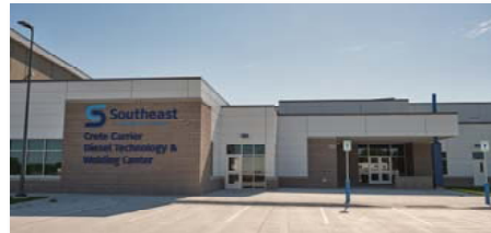
Crete Carrier Diesel Technology & Welding Center, Milford
